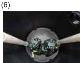
(6) Pump orientation, tie the cord with strip.
