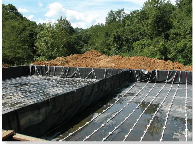
Large-capacity Z-Cell upflow wetland under construction.
