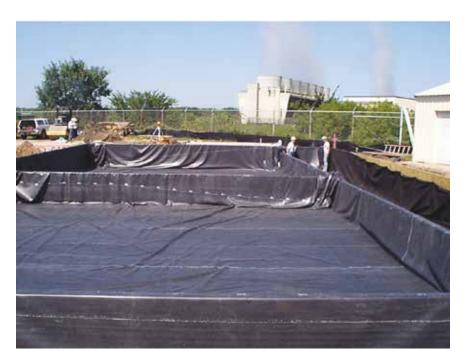
Zoeller Pump Company EPDM liners provide a superior barrier to flexible PVC in applications such as recirculating media filters, constructed wetlands and ponds. Custom sizes are available.
