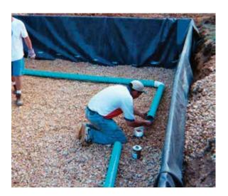
Zoeller Pump Company's EPDM liner is a very effective way to make in-ground treatment installations, such as recirculating media filters and constructed wetlands, watertight. Zoeller Pump Company provides custom sizes and the expertise to work with and service liners in the field. Accessory items such as pipe boots, splice kits, and repair kits are also available. Made from EPDM rubber, the 45 mil liners are stronger, more durable, and more chemically stable than their flexible PVC counterpart.
