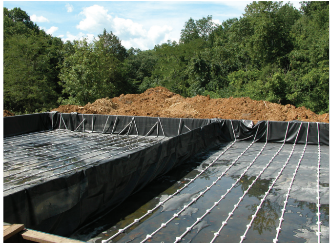
Large-capacity Z-Cell upflow wetland under construction.
