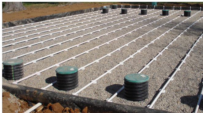
Partially constructed recirculating media filter
